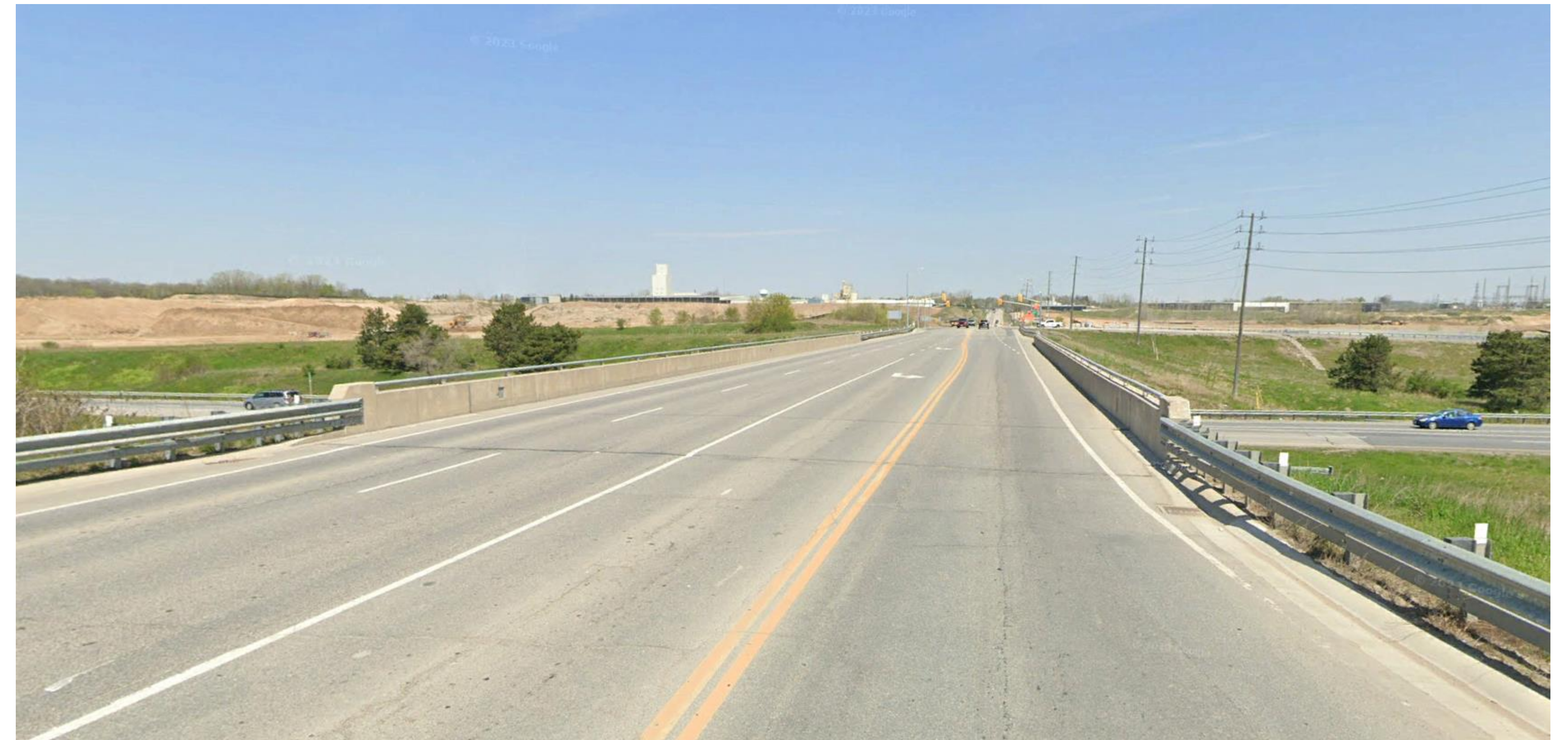
Oak Park Road at overpass bridge over Highway 403, looking north
