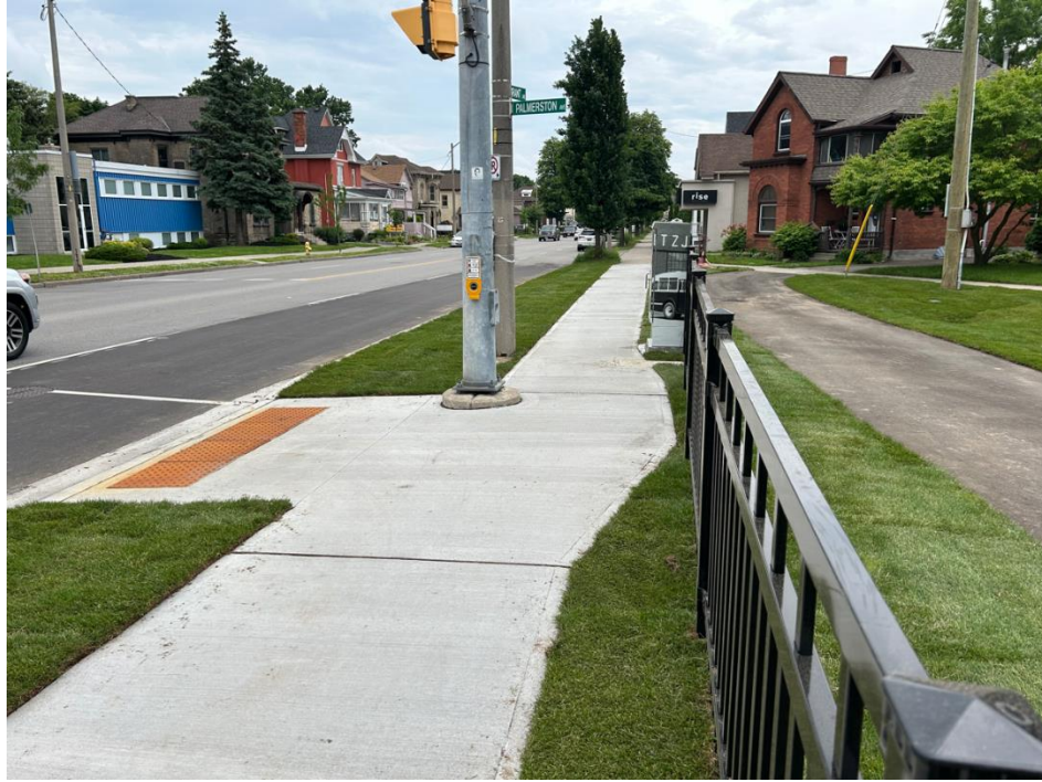
Figure 2 - Palmerston Street and Brant Avenue New Sidewalk and Tactile Walking Surface Indicators
