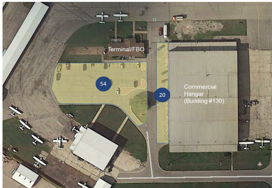
Exhibit 6-2 – Existing Airport Terminal/FBO Parking Lot
